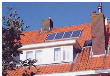
Example of a solar station with four 120Wp solar panels, suitable for Soladin peak capacity: 480Wp. Energy saving, depending on usage, up to 12%.
